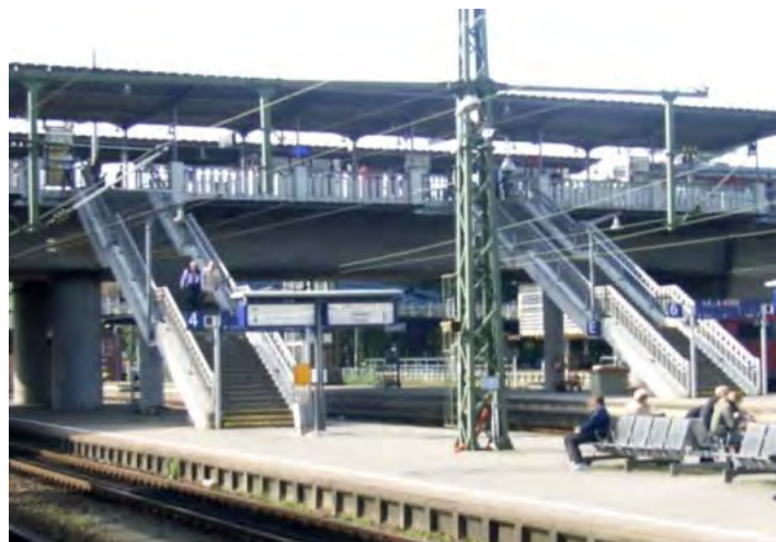
Fig. 13: Direct access from trams to trains in Freiburg
